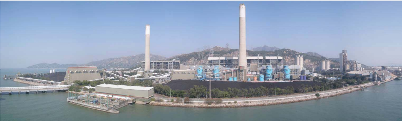
Overview of Castle Peak Power Station after retrofit of EC facilities
